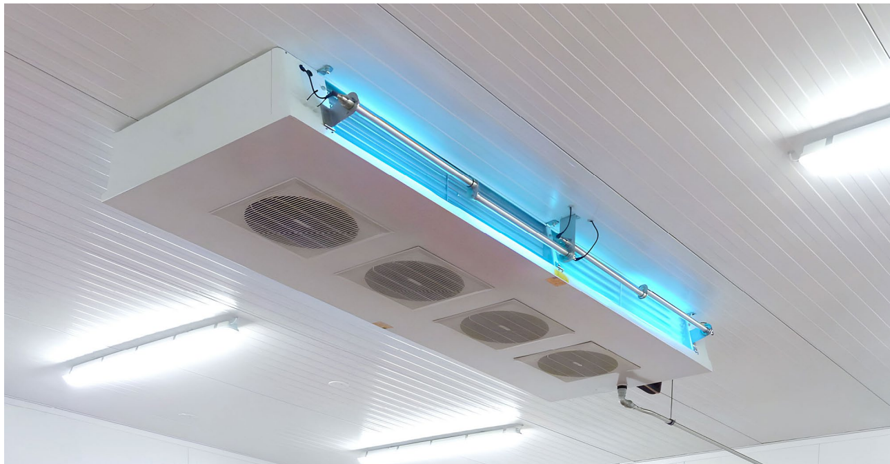
UVC units installed in front of evaporator fins prevent the formation of biofilm and contamination of ambient air.
